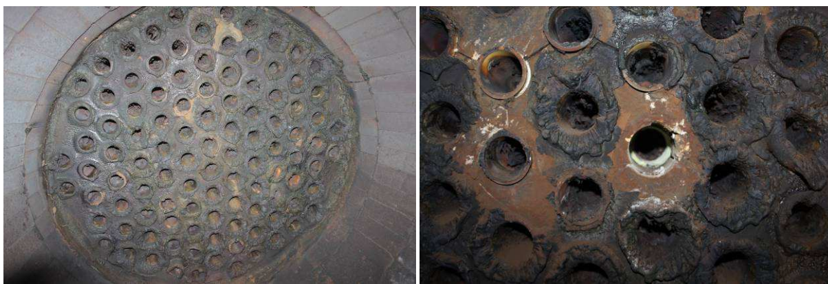
Photo 2. Smoke tube with deposits restricting flu gas flow to the boiler 1 st pass.
