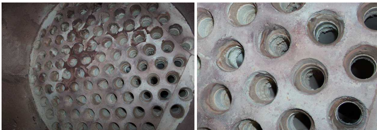
Photo 11. Additional cleaning effect using shock wave. The first pass outlet tube sheet with no deposits restricting flue gas flow.
