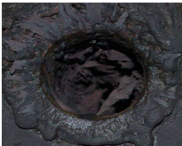
Photo 3. Fouled smoke tubes in the heat recovery boiler first pass.
