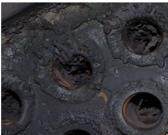
Photo 3. Fouled smoke tubes in the heat recovery boiler first pass.
