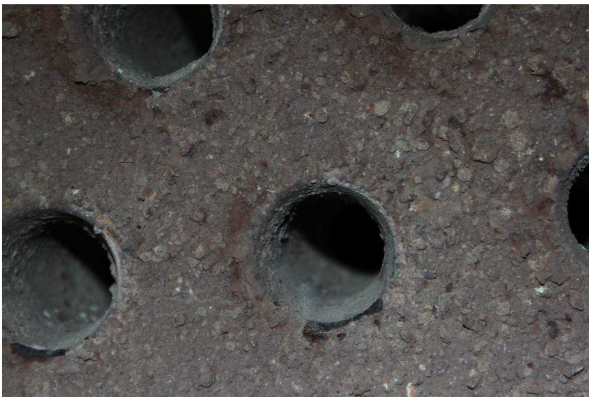
Photo 10. Smoke tubes with no fine deposit at all.
