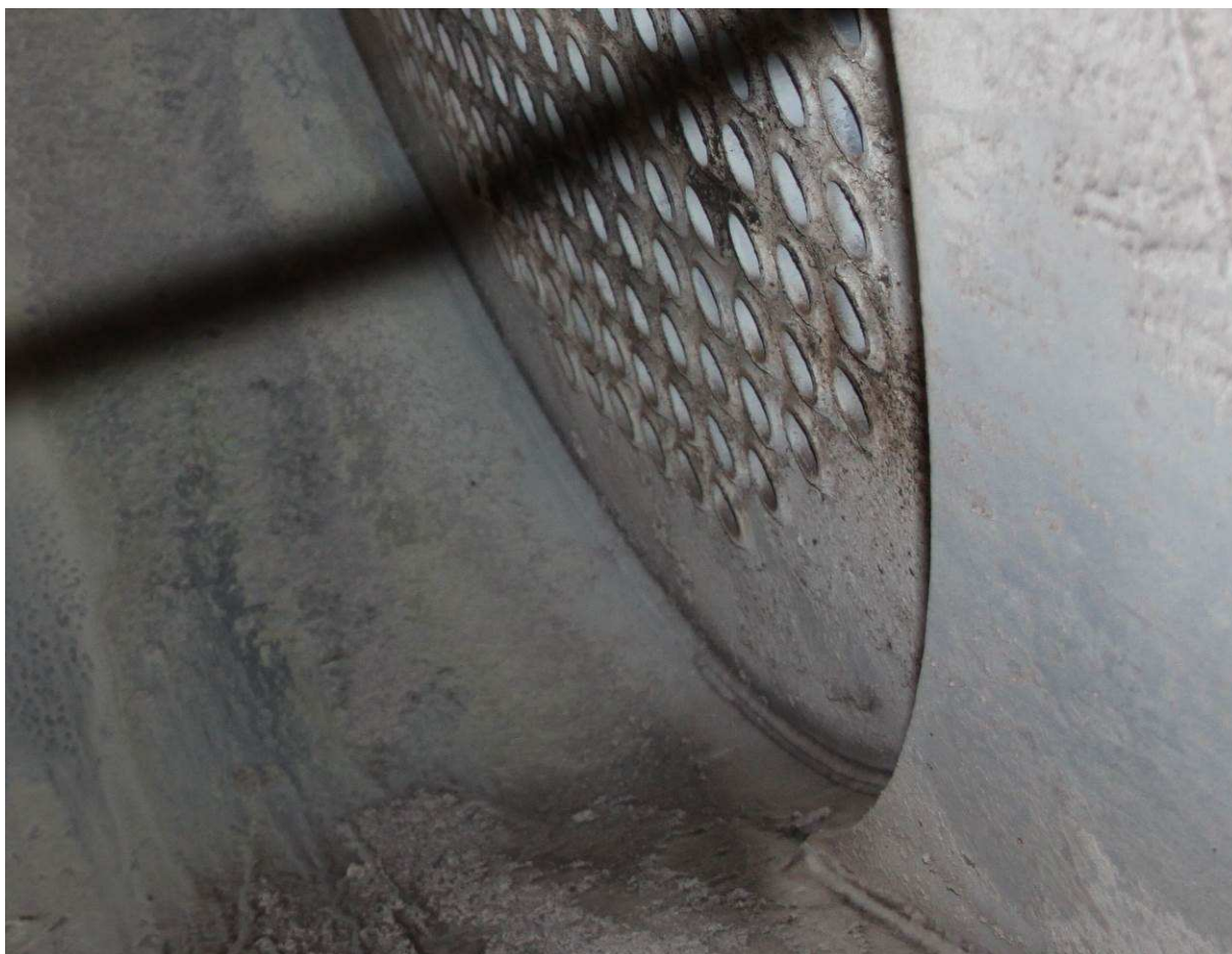
Photo 15. The flue gas outlet header downstream the heat recovery boiler with visible two inlets of the shock wave.
