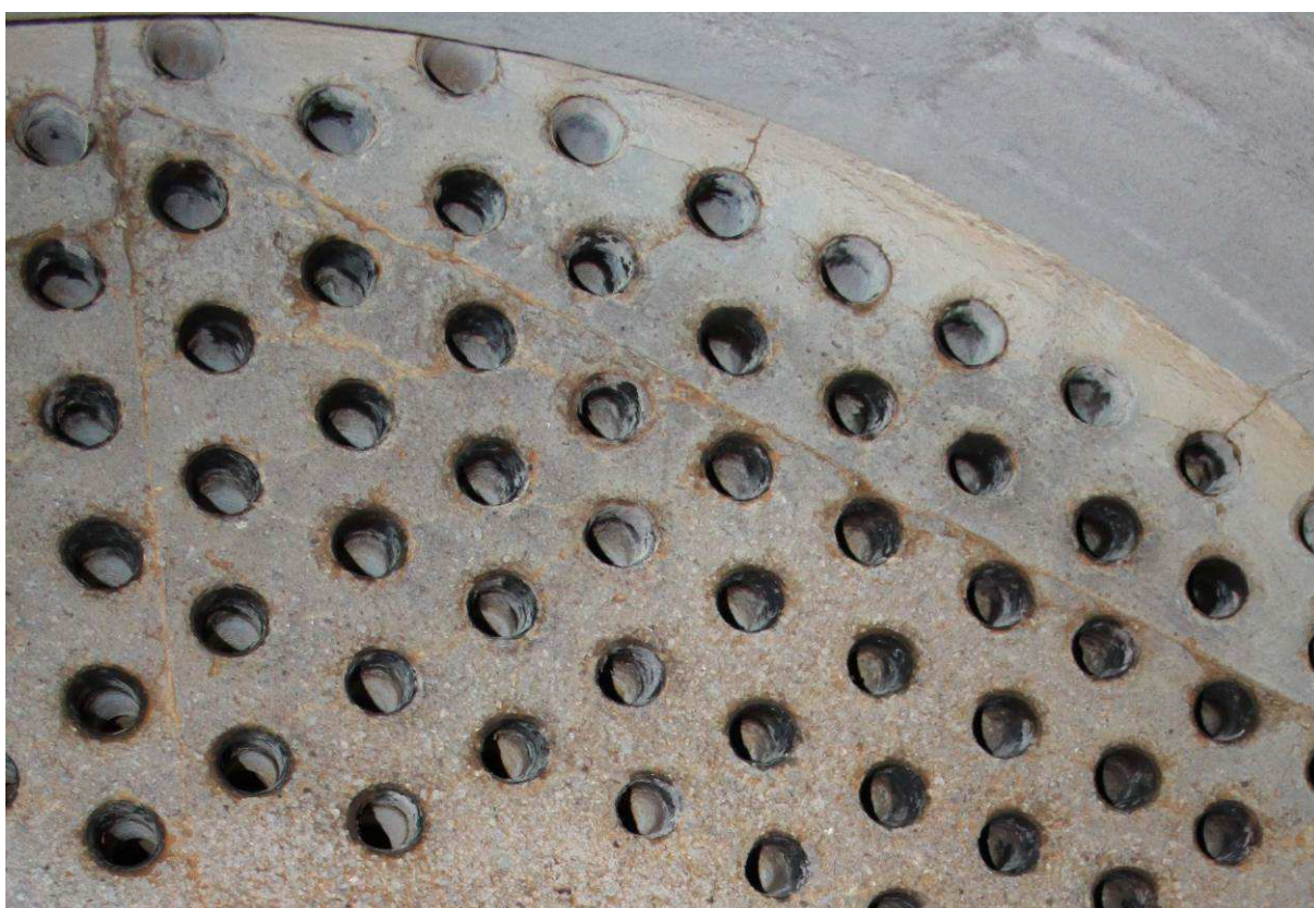
Photo 12. Upper part of the second pass tube sheet with no fine deposits at all.
