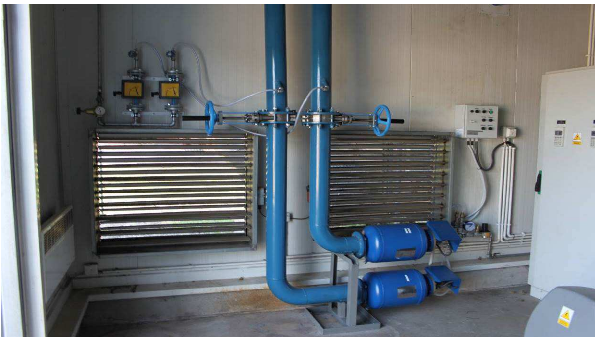
Photo 7. Two GFU-24/8 shock wave generators, located in the electrostatic precipitator room.
