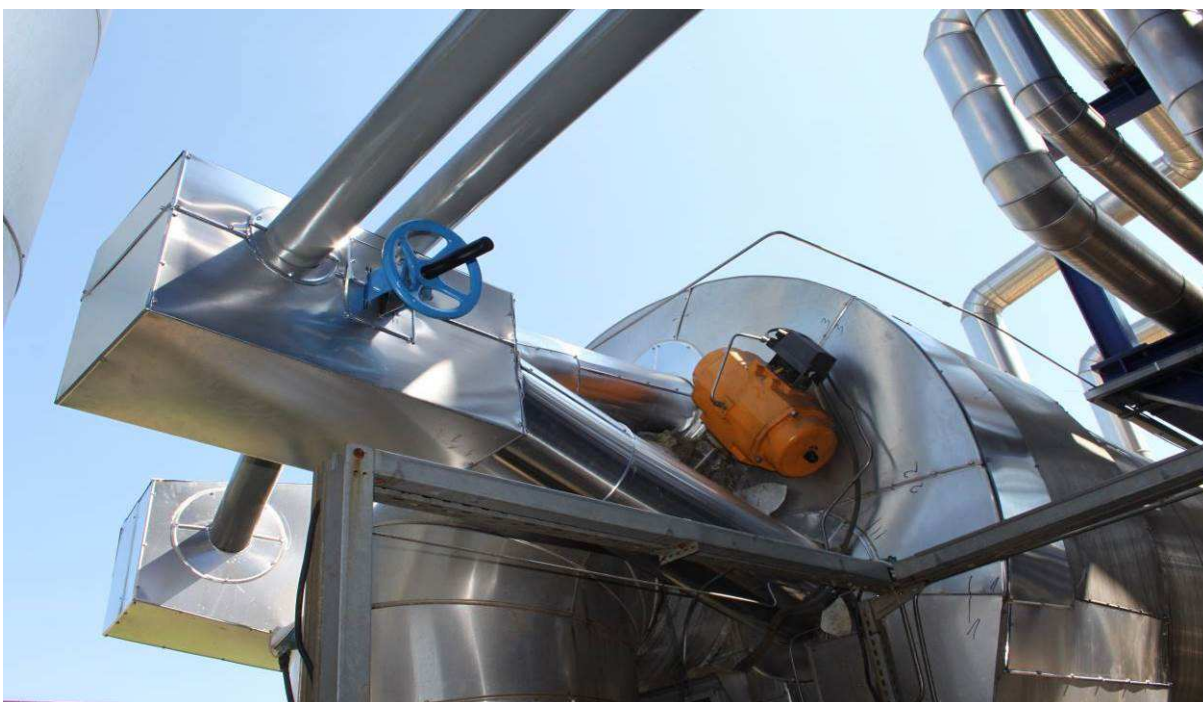
Photo 8. Shock wave inlet for smoke tube cleaning.
