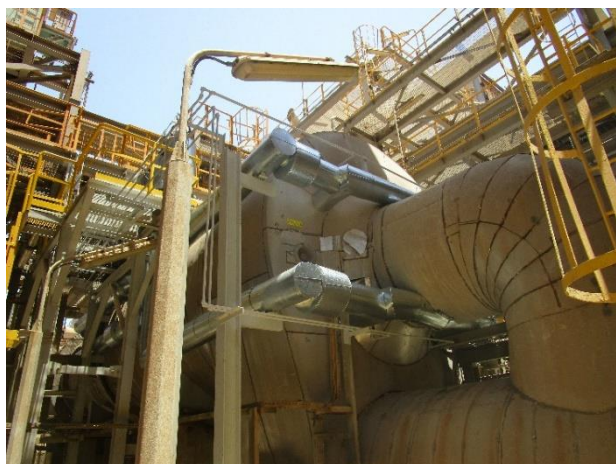
Cleaning installation of waste heat boiler (pipelines covered with galvanized sheet) – TASNEE Saudi Arabia
