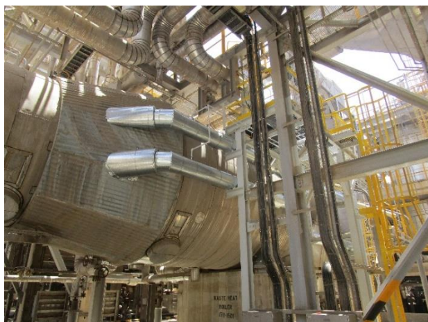
Cleaning installation of waste heat boiler (pipelines covered with galvanized sheet) – TASNEE Saudi Arabia
