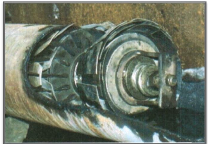
Introduction of the generator to the pipeline
