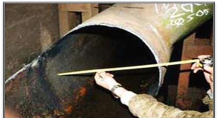
The pipe after cleaning using a cavitation generator
