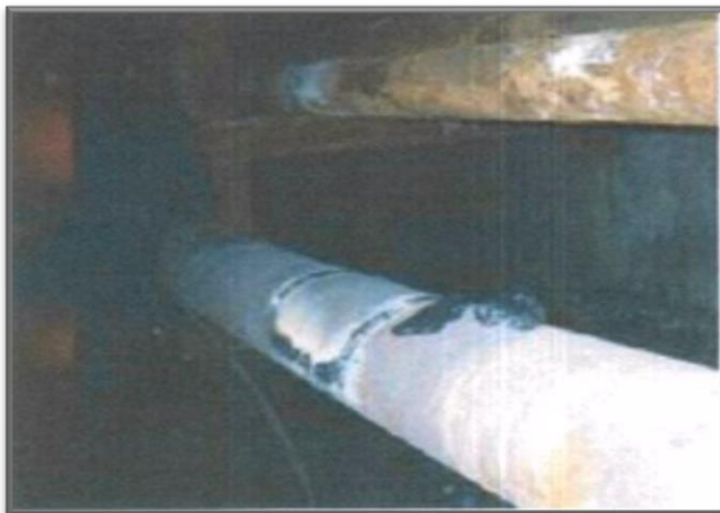
Blanking of the inspection hole and activation of pressure pumps
