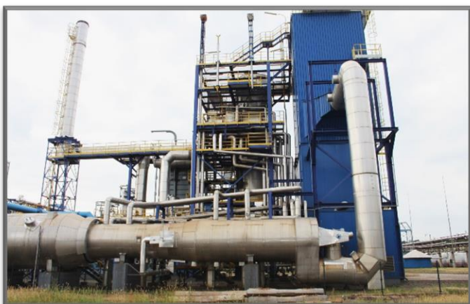
Petrochemia Blachownia S.A – installation of liquid waste disposal
